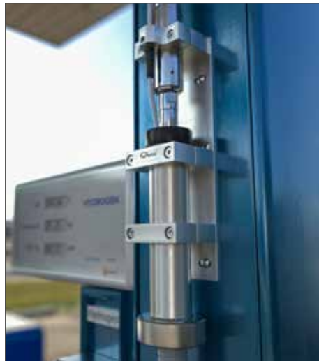
WEH® TSA1 CNG Breakaway Coupling
