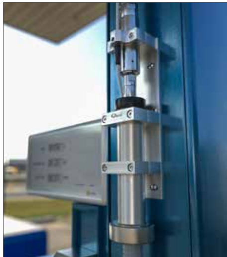
WEH® TSA1 H 2 70 MPa Breakaway Coupling
